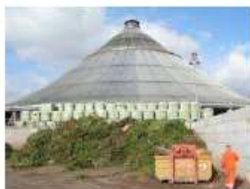
waste treatment plant „Rinterzelt“
